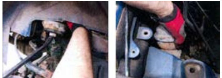
Figure 17-18: Lift out the displacer through the engine bay, rather than the wheel arch.
